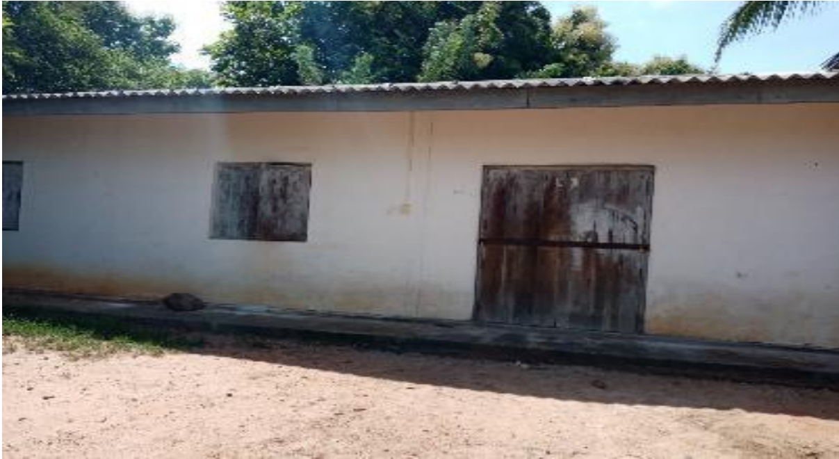
Old building side view
